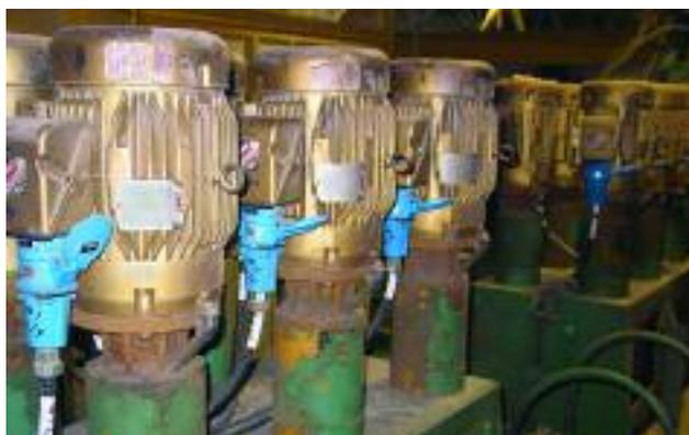
*Decontactors enable quick motor change-outs*
